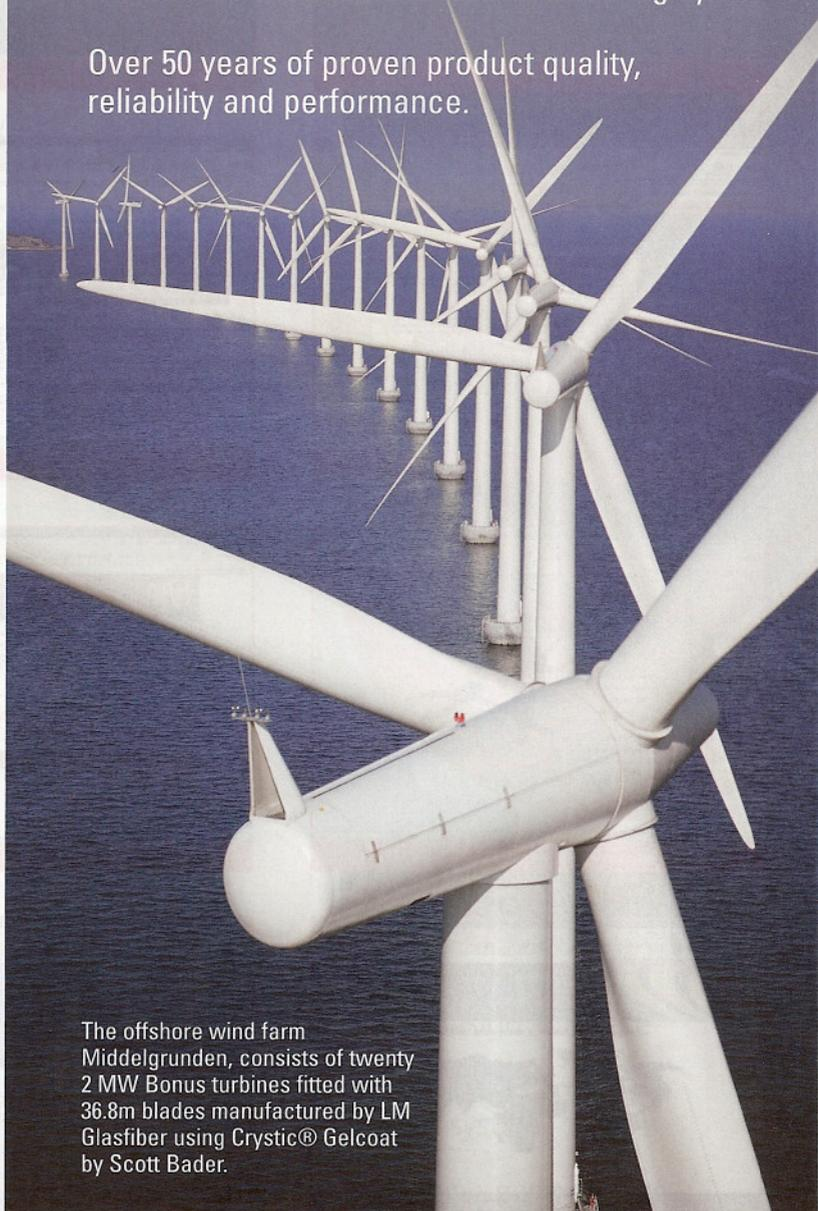
The offshore wind farm Middelgrunden, consists of twenty 2 MW Bonus turbines fitted with 36.8m blades manufactured by LM Glasfiber using Crystic® Gelcoat by Scott Bader.
